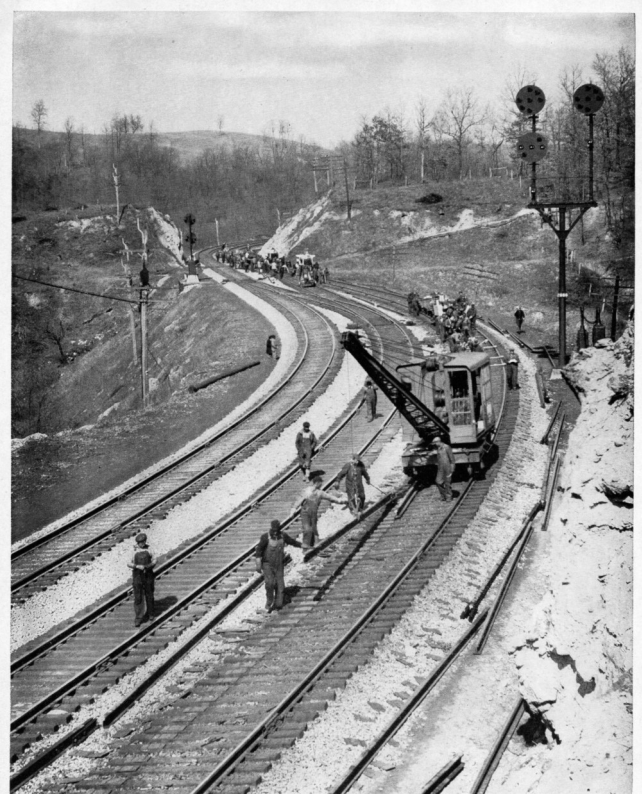
The Track Repairmen at Work
