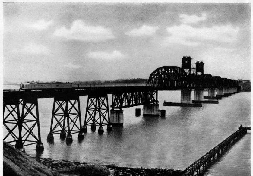
A Train Crossing a Bridge
