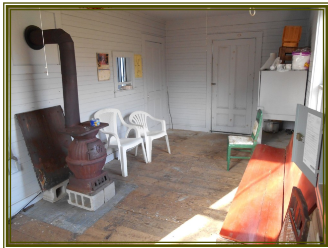
Figure 3A – Current Station Waiting Room – Photo Courtesy of WW&F Ry Museum – I am sure the plastic chairs weren't part of the original 1925 furniture!
