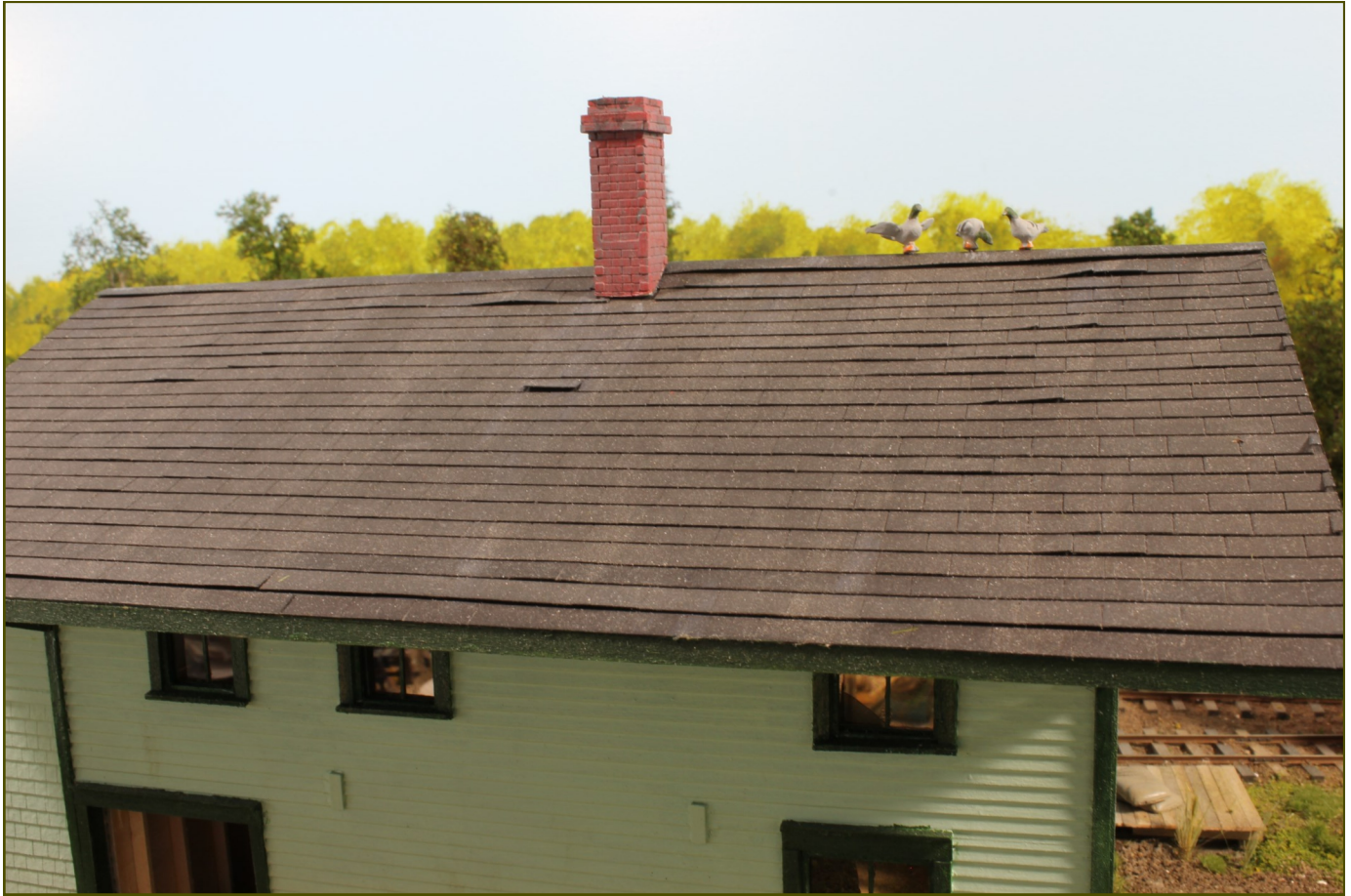
5 - Paper Shingles Installed on Albion Station
